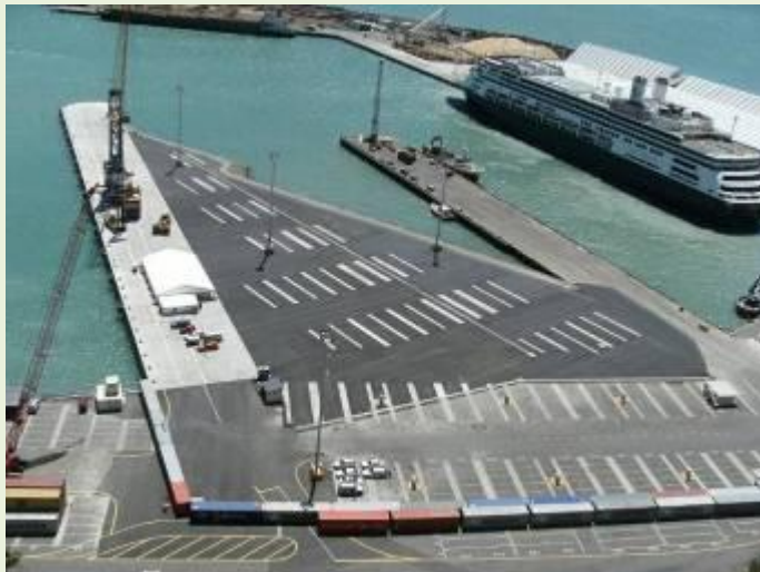
New $47 million wharf opened at the Port of Napier last Friday
